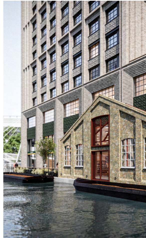
View of new canal side path, showing retained warehouse façade
