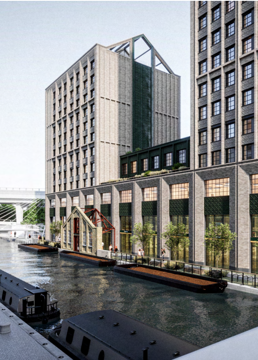
View of new canal side path, showing retained warehouse façade
